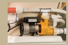
**Powerful Pump Motors** A powerful 7.8 amp motor is standard on all PROFLO PLUS whirlpool baths. The pump motor is pre-wired and preplumbed for simple plug-in installation. Requires a single 115V/20 amp GFCI circuit.
