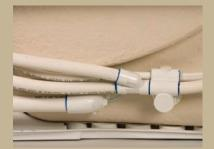
Water Tested Plumbing Each joint is solvent welded and water tested prior to delivery for long-term reliability.
